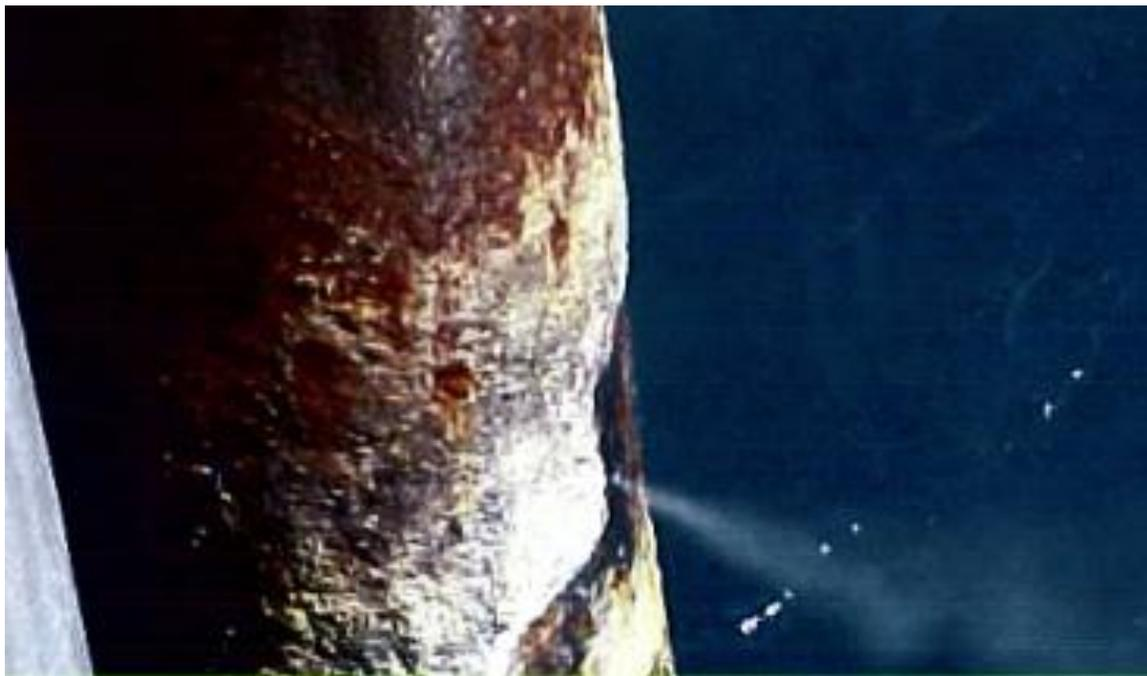
Figure 1 – gas leak from conductor
